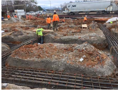
Excavation Work Correct Excavation Shoring?
