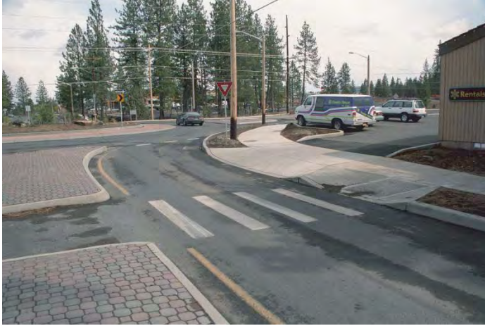
(a) Driveway between crosswalk and roundabout (Bend, Oregon)
