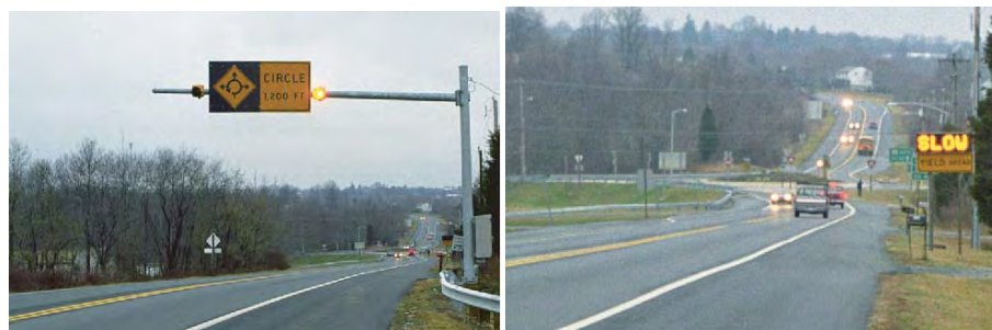
(a) Warning beacons (Leeds, Maryland) (b) Dynamic speed warning signs (Leeds, Maryland)
