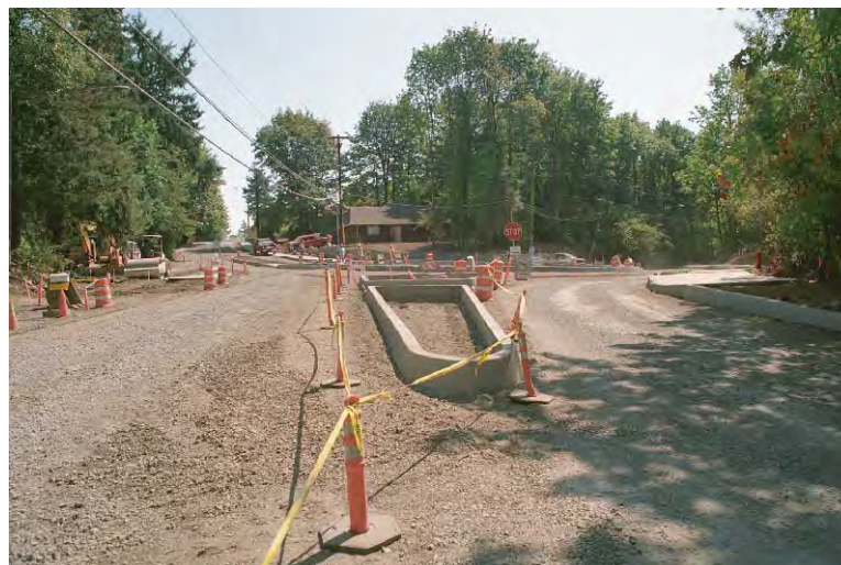
(a) Splitter island construction (Portland, Oregon)
