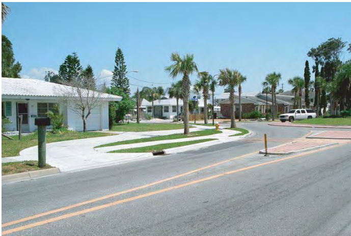
(c) Driveway reconfiguration (Clearwater, Florida)
