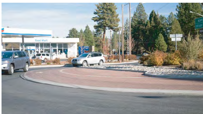
(b) Maintenance pullout in central island (Bend, Oregon)
