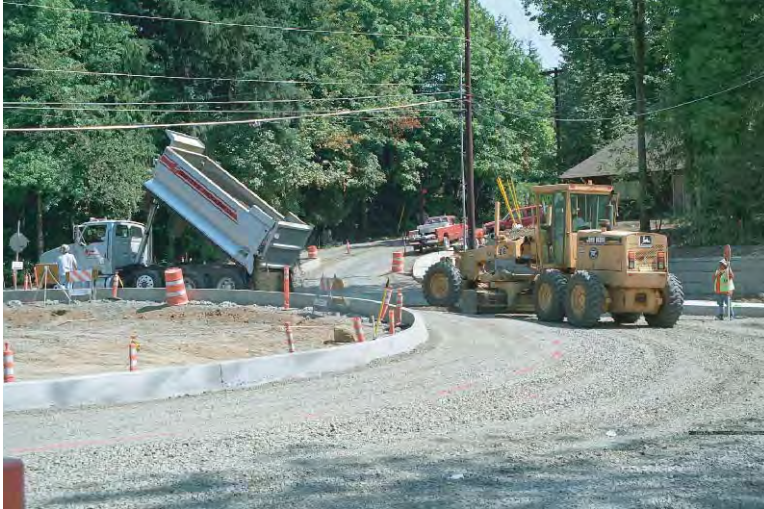
(b) Circulatory roadway sub-grade construction (Portland, Oregon)
