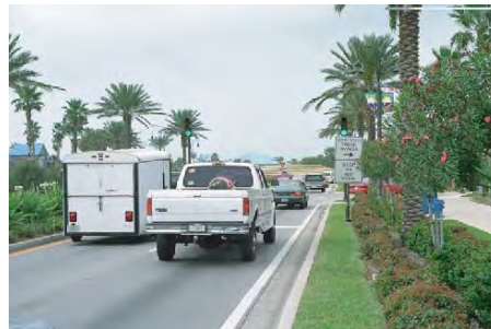
(a) Approach metering signal Clearwater, Florida
