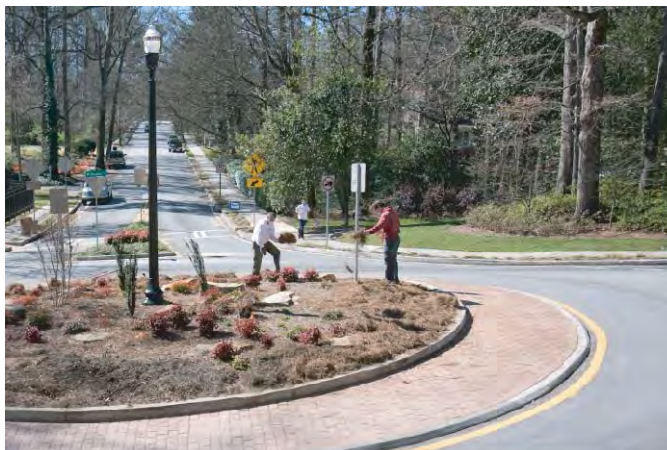
(a) Central island maintenance (Decatur, Georgia)
