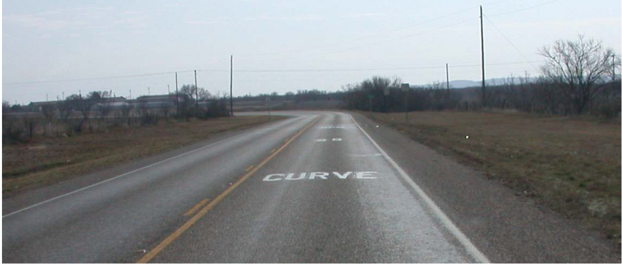
Figure 3.18 Text and advisory speed horizontal signing applications (39).
