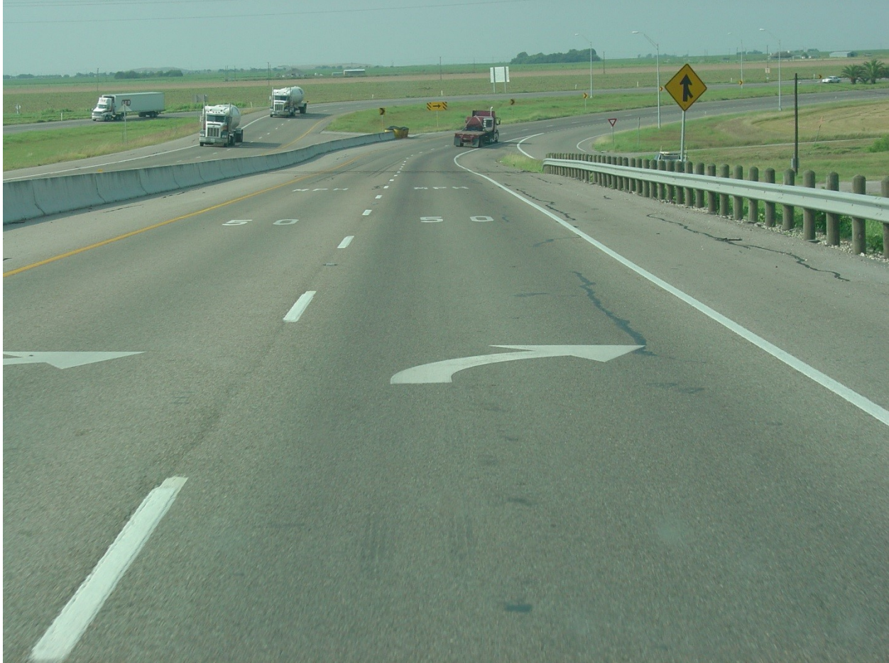
Figure 3.19 Urban freeway curve warning pavement markings (39).
