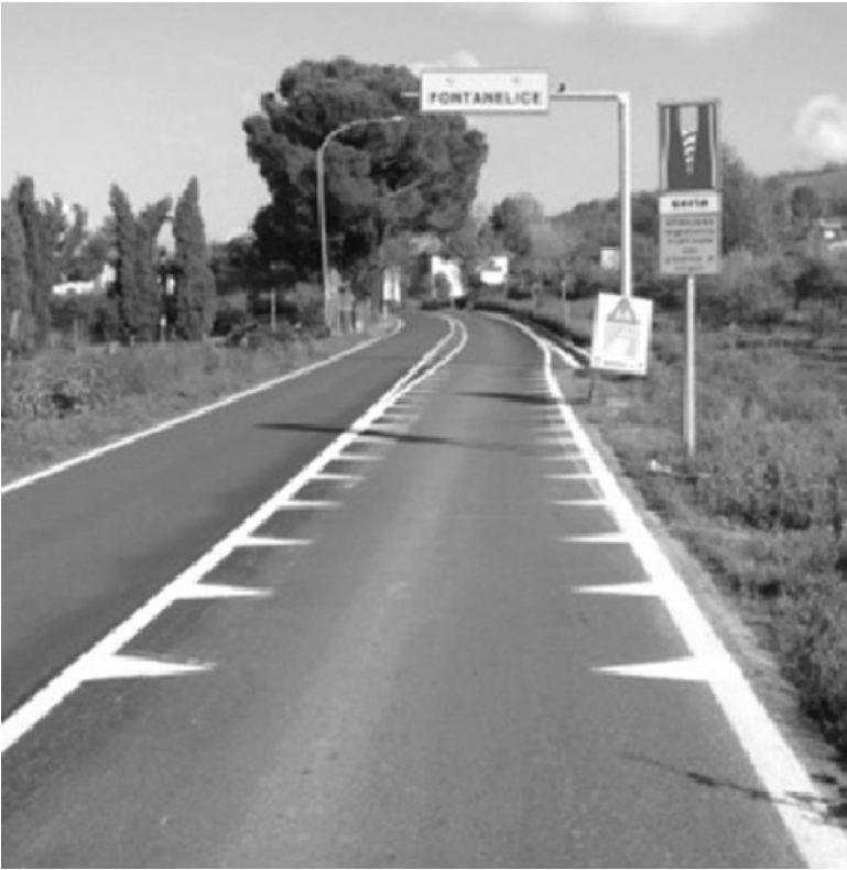
Gateway treatment in Italy transitioning from rural road to village. Source: Lantieri, C., Lamperti, R., Simone, A., Costa, M., Vignali, V., Sangiorgi, C., & Dondi, G. (2015). Gateway design assessment in the transition from high to low speed areas. Transportation Research Part F: Traffic Psychology and Behaviour, 34, 41-53.
