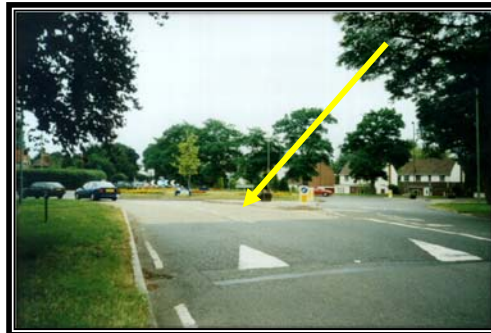
Raised crosswalk at roundabout in the UK
